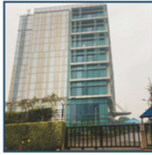
Uniworld Commercial Tower
