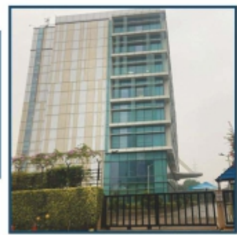
Uniworld Commercial Tower
